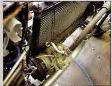
With these heavy-duty zip ties in place, the A/C compressor is well out of the way for installing the new engine.
